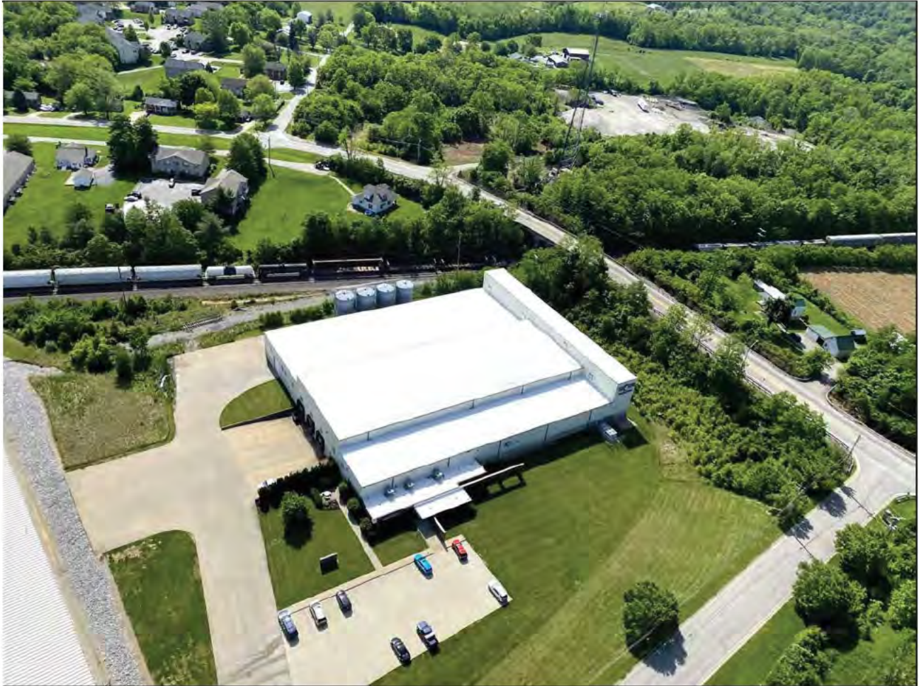
View facing generally east and showing the US-25 underpass. Crittenden, Grant County, KY
