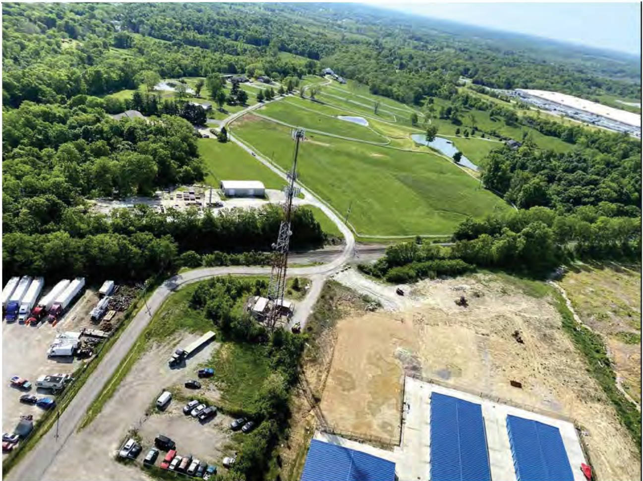
South of Florence, KY at the Totten Lane crossing. Boone County, KY
