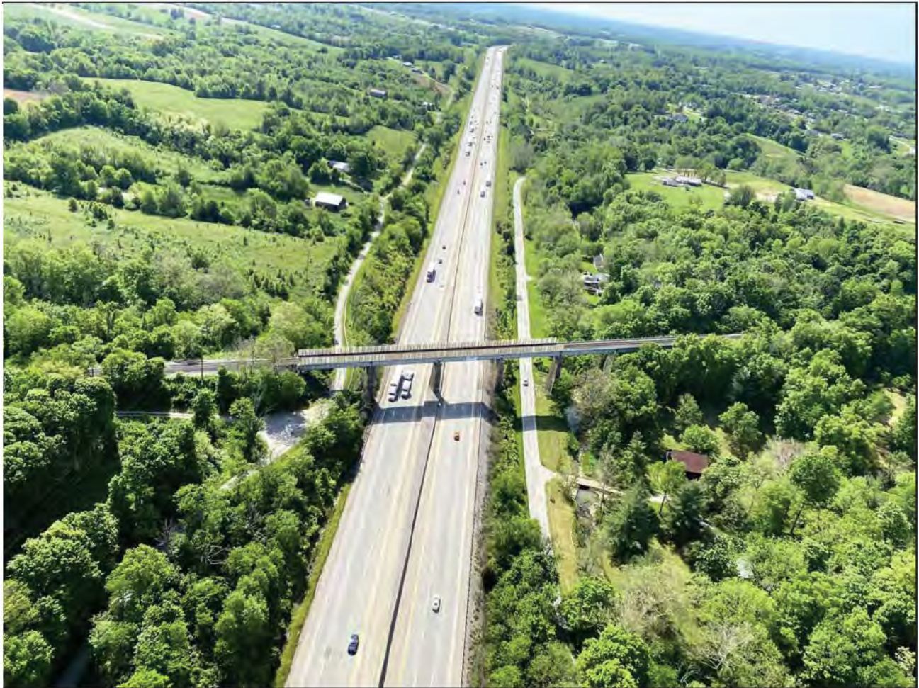
Rail bridge over Interstate 75, South of Walton, Boone County, KY
