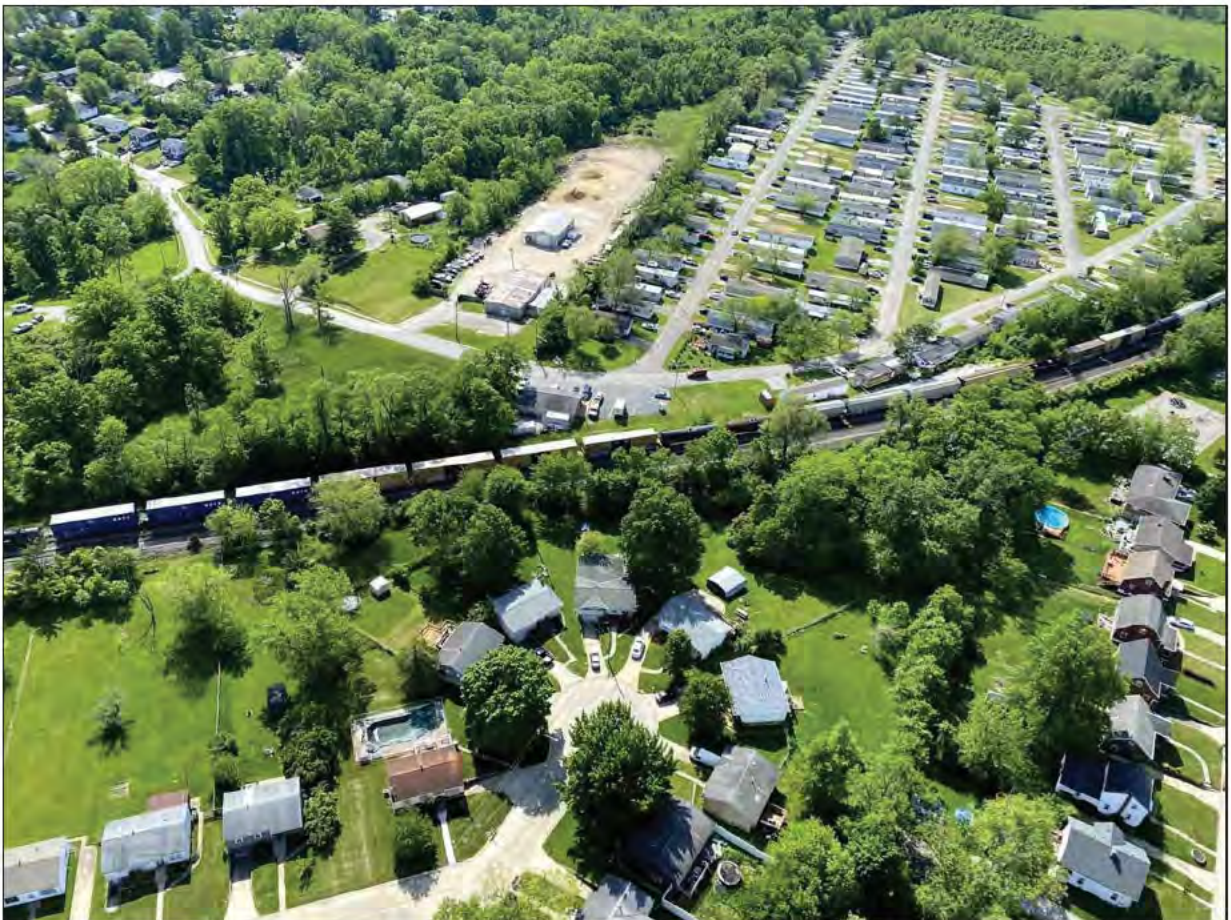
Typical subject view taken facing southeast. Elsmere, Kenton County, KY
