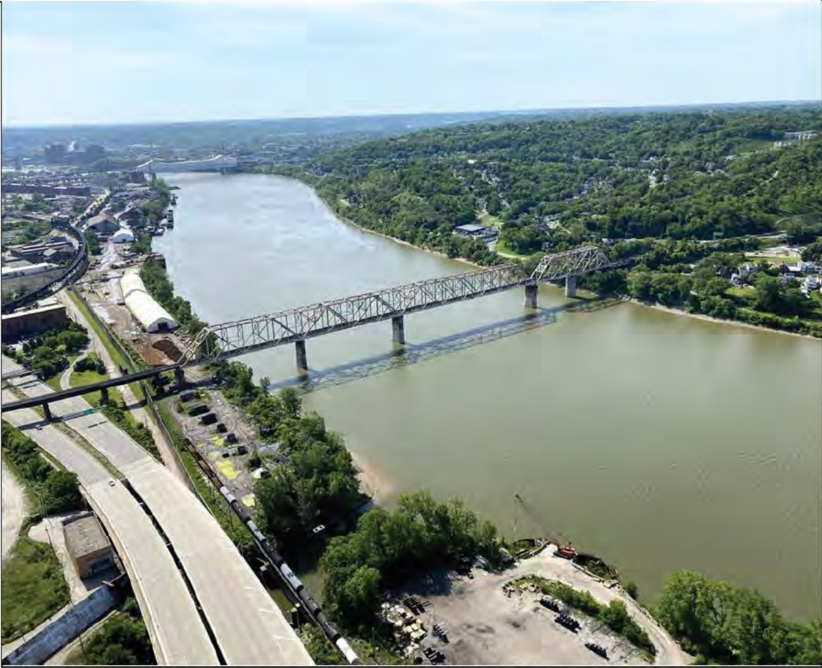
View of the rail bridge over the Ohio River facing east/southeast, Highway 50 to the left
