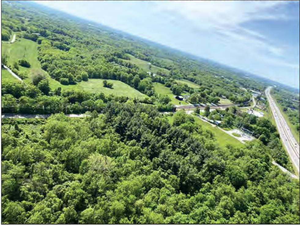
Grant County, KY facing south/southeast - I-75 to the right
