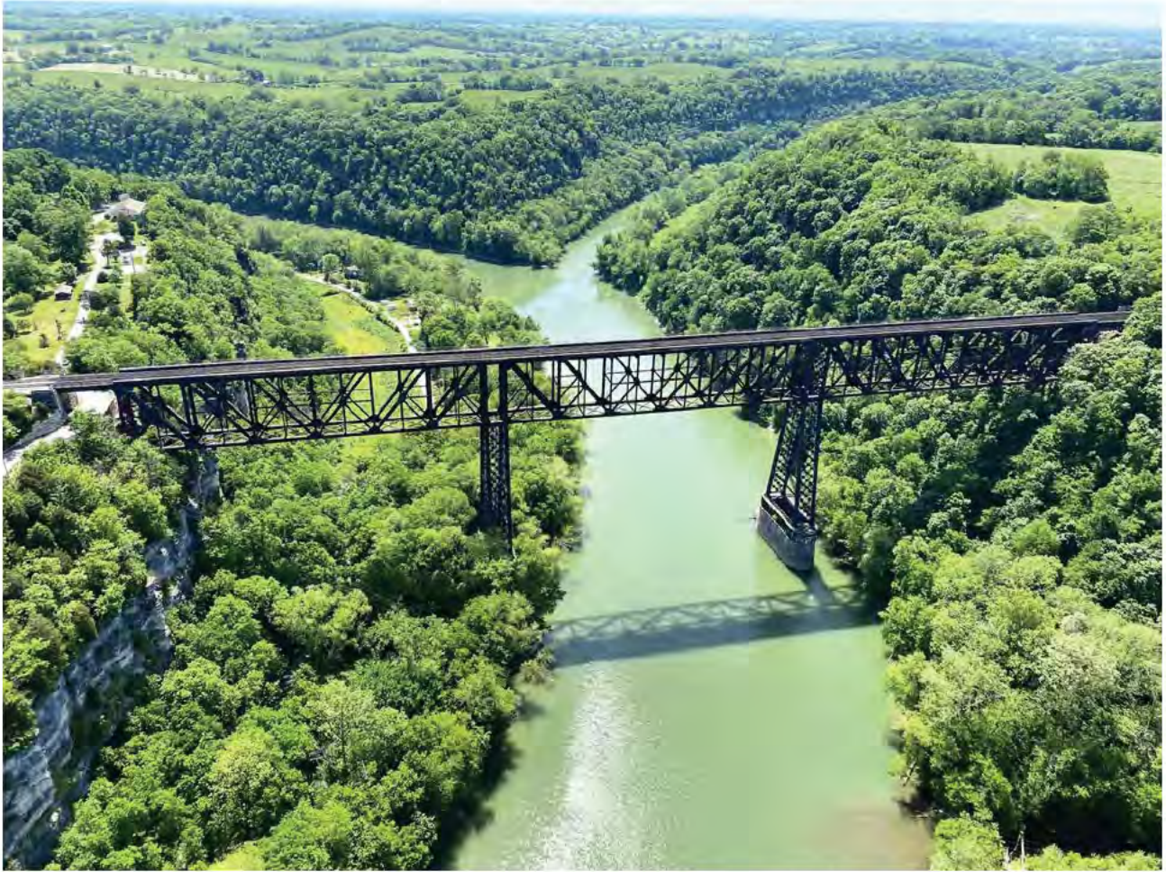
View of High Bridge over the Kentucky River, Jessamine County, KY
